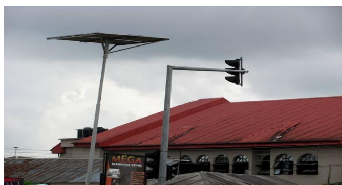
Fig. 6. Solar powered traffic light in Nigeria.
